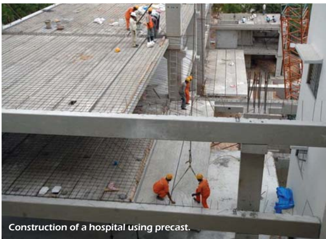
Workers lower a panel into position.
