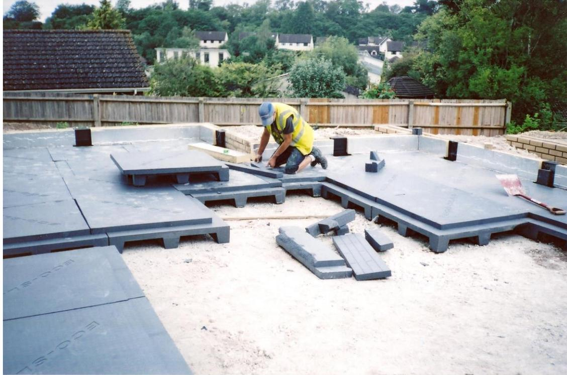
Figure 1 Placing the insulation units.
