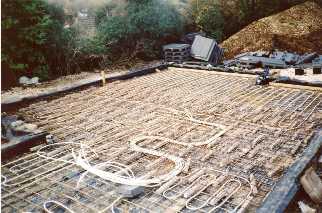
Figure 2. Typical example of the reinforcement and underfloor heating pipe layout.
