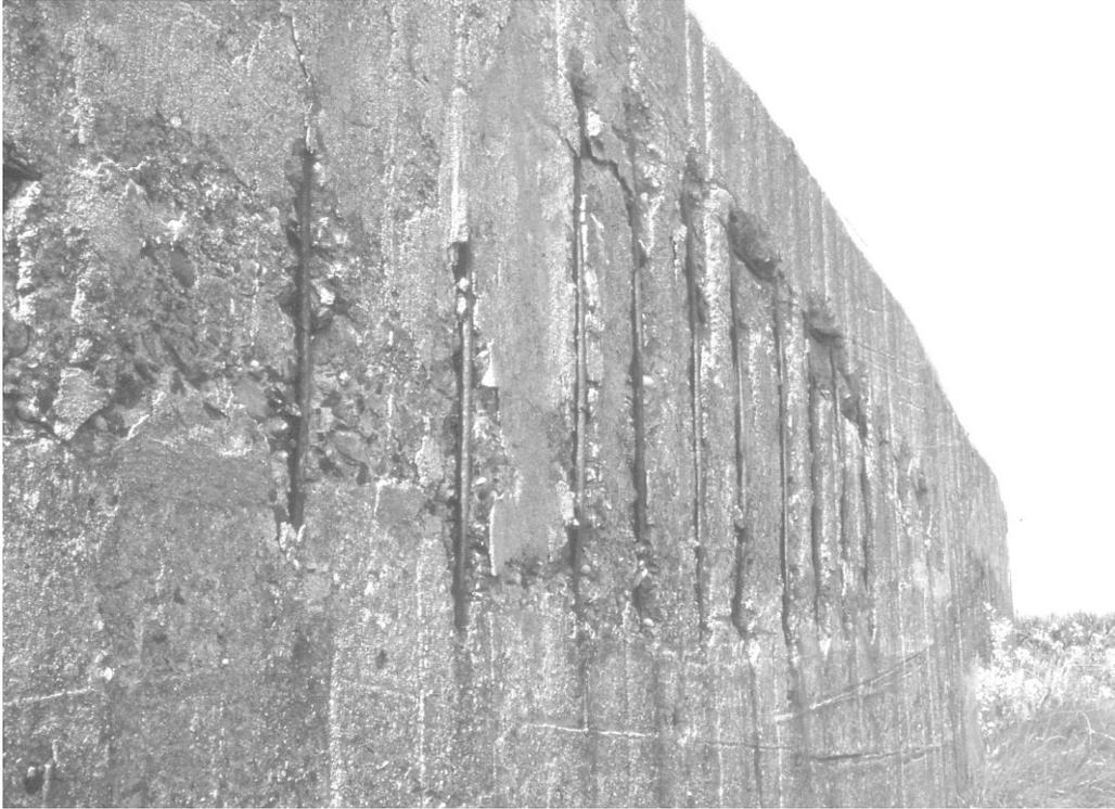
Figure 1. Example of corroded reinforcement resulting from the failure to achieve the specified cover.
