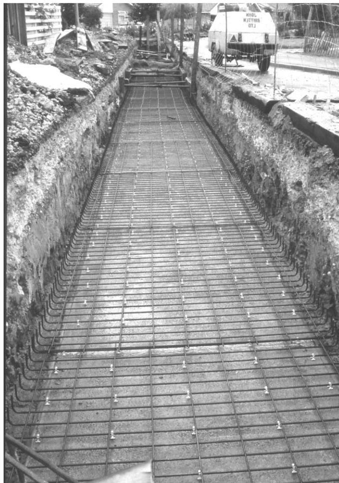
Figure 2. Example of spacers being fixed in accordance with BS7973 for the roof of a culvert built using permanent formwork and pre-bent fabric.
