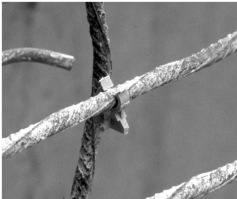
Figure 3. Reinforcement in-situ with spacer still attached.
